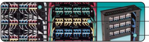
Vertical cable management enables easy, quick addition and removal of patch cords while effectively retaining them through the channel
